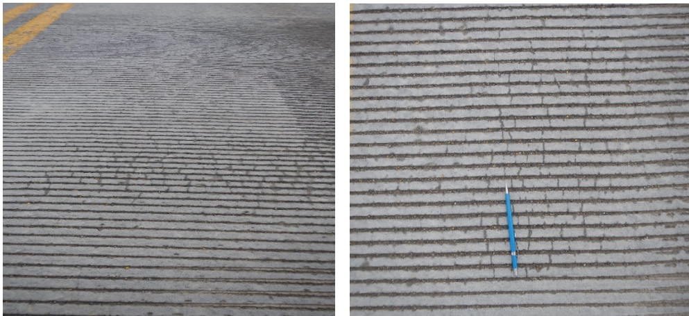
Figure 11: Shoup Bridge – 17 months Bridge Deck Cracking Survey, random fine crazing cracks parallel to span length (All photos provided by FHWA Federal Lands)
