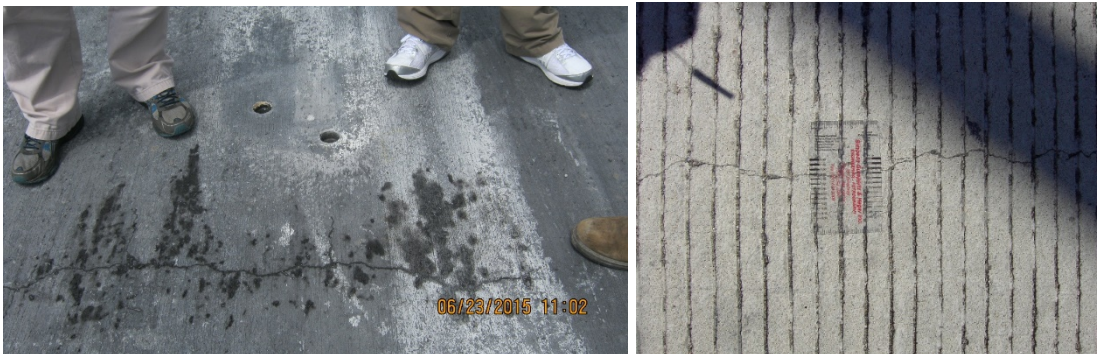
Figure 1: Examples of Bridge Deck Cracking (All photos provided by FHWA Federal Lands)
