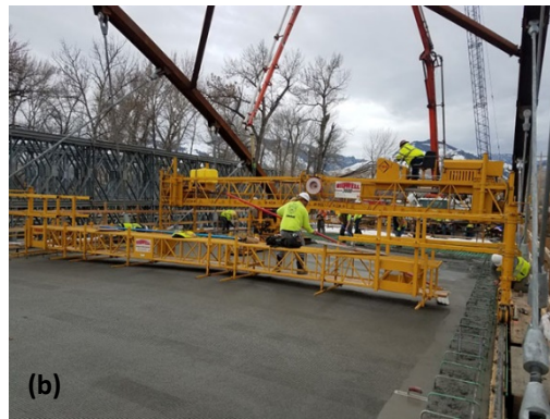
Figure 4: Initial Use of Pump Ft. Pulaski changed to 3 Yard Hopper Dump (All photos provided by FHWA Federal Lands)
