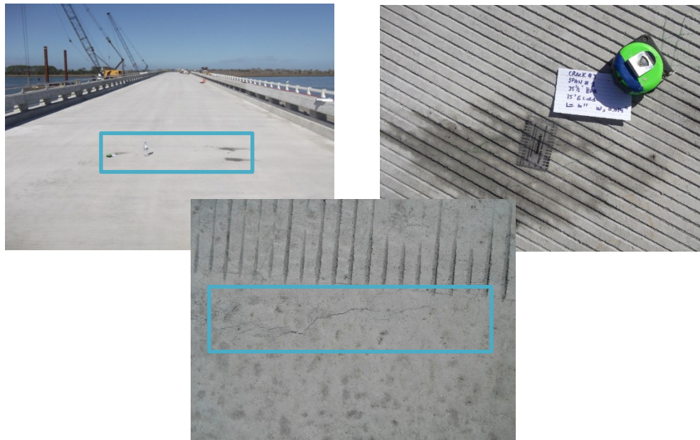
Figure 14: Ft Pulaski – 3 and 14 months Bridge Deck Cracking Survey, cracking on span 1 (All photos provided by FHWA Federal Lands)
